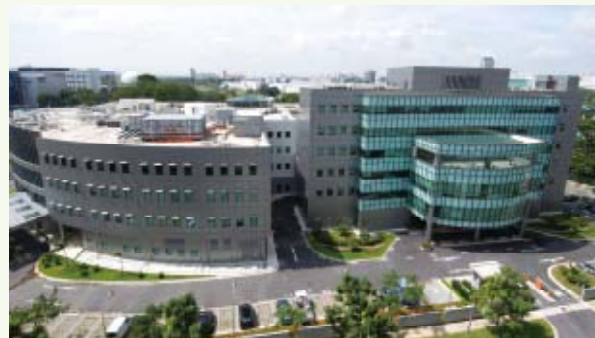
Exterior View of WaterHub
