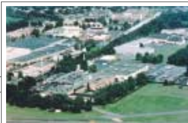
New Brunswick plant (New Jersey, USA)
