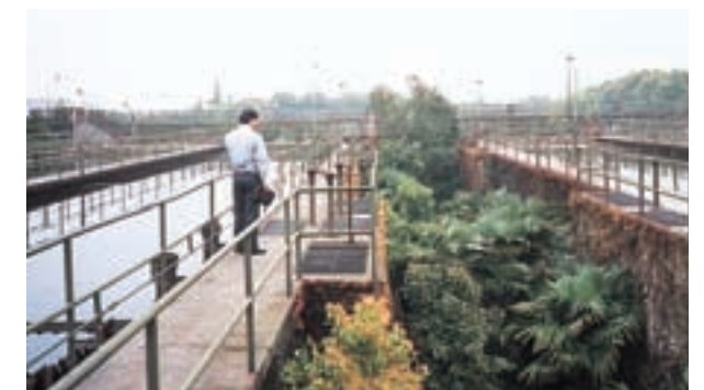
Industrial park wastewater treatment facilities in Shanghai
