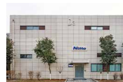
Building exterior, Nitto (Qingdao) Technology Research Institute
