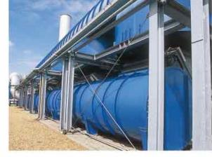
The new deodorizing furnace is a regenerative furnace, which does not require energy supply from outside during its operation. The collected thermal energy is used not only to operate the equipment itself but also to supply steam and coolant to the production process and heat to the building.
