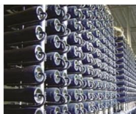
Reserve osmosis membrane modules for seawater desalination system
