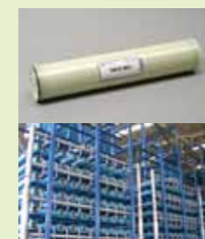
Reverse Osmosis Membrane Module
