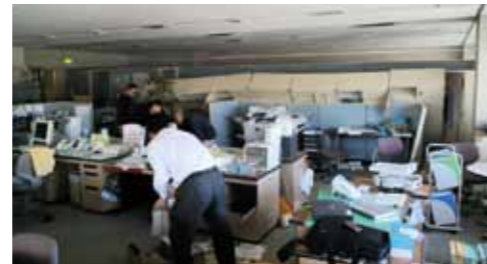
Office of Nitto Denko Tohoku Sales Branch in Sendai-shi The cabinet was fixed to the wall but fell because of the violent shaking of the earthquake.
