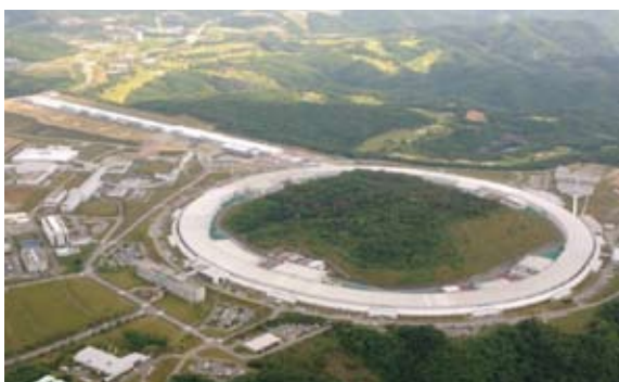
An aerial view of the SPring-8 large-scale synchrotron radiation facility © RIKEN/JASRI
