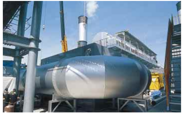
New deodorizing furnace under construction at the Onomichi Plant
