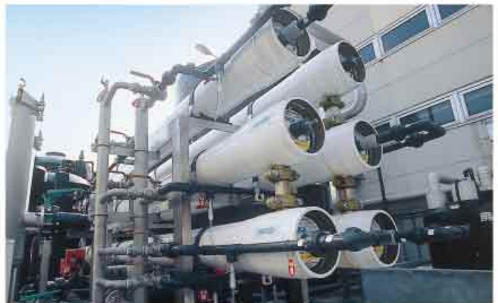
The Nitto Denko Group seawater desalting membranes are producing about 1 million m 3 of desalinated freshwater each day
