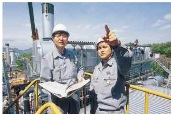
In front of Deodorizing furnace under construction
