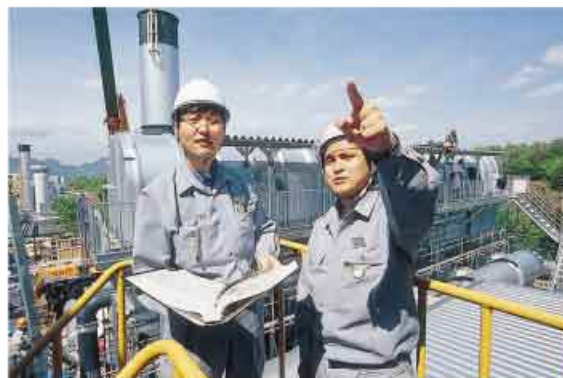
In front of Deodorizing furnace under construction
