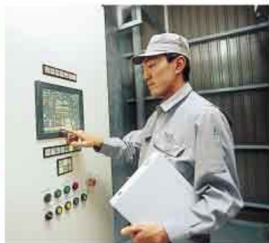
Deodorizing furnace of factory No.9, Kameyama Plant
