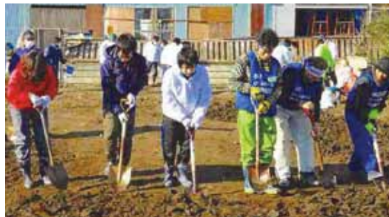
Leveling of land
