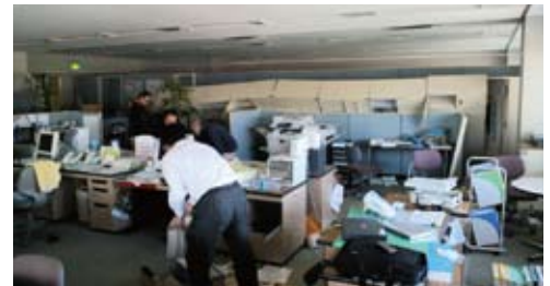
Office of Nitto Denko Tohoku Sales Branch in Sendai-shi The cabinet was fixed to the wall but fell because of the violent shaking of the earthquake.
